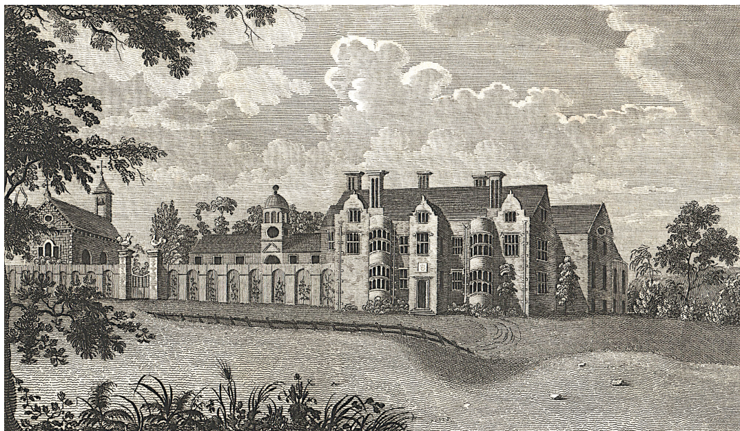
Fig. 7. Glyde Place, Glyde, c1780; John Morris built the bow windows, the screen wall and the church and designed and built the stables (© Sussex Archaeological Society).
